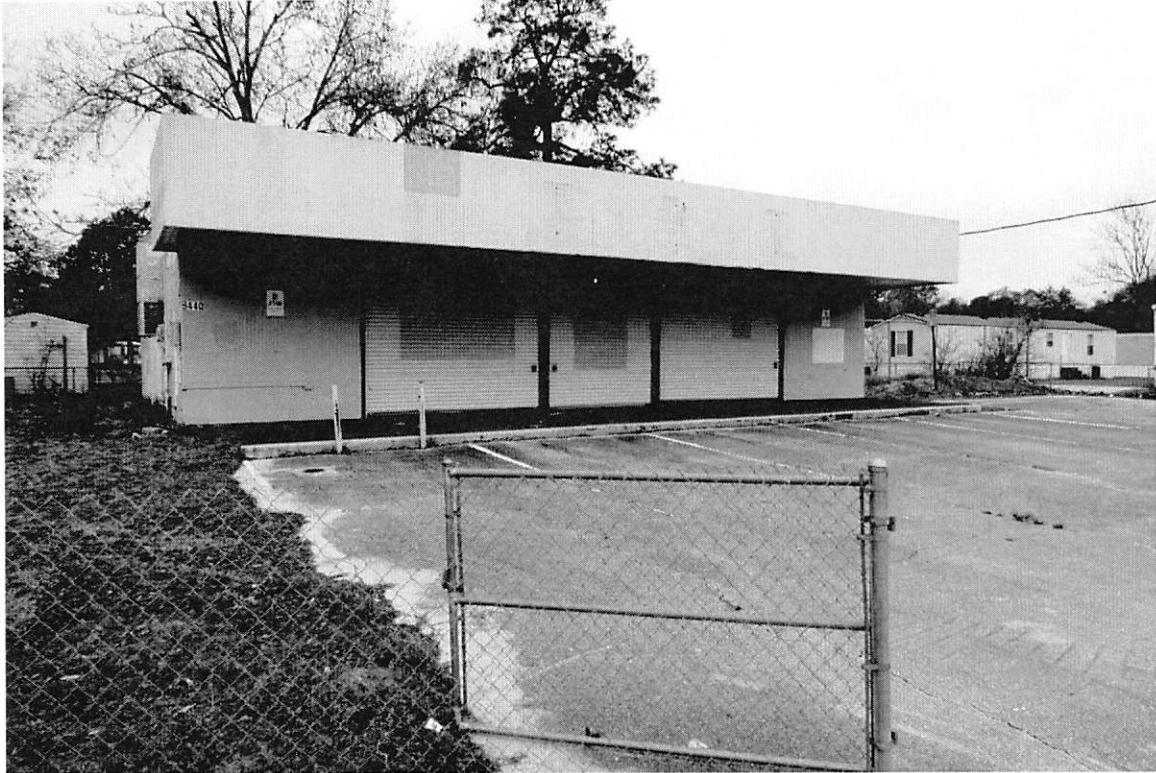
View of existing building
